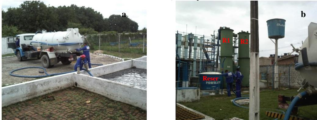
R1: reator UASB; R2: reator Híbrido; Reser: reservatório de 3 m<sup>3</sup>
