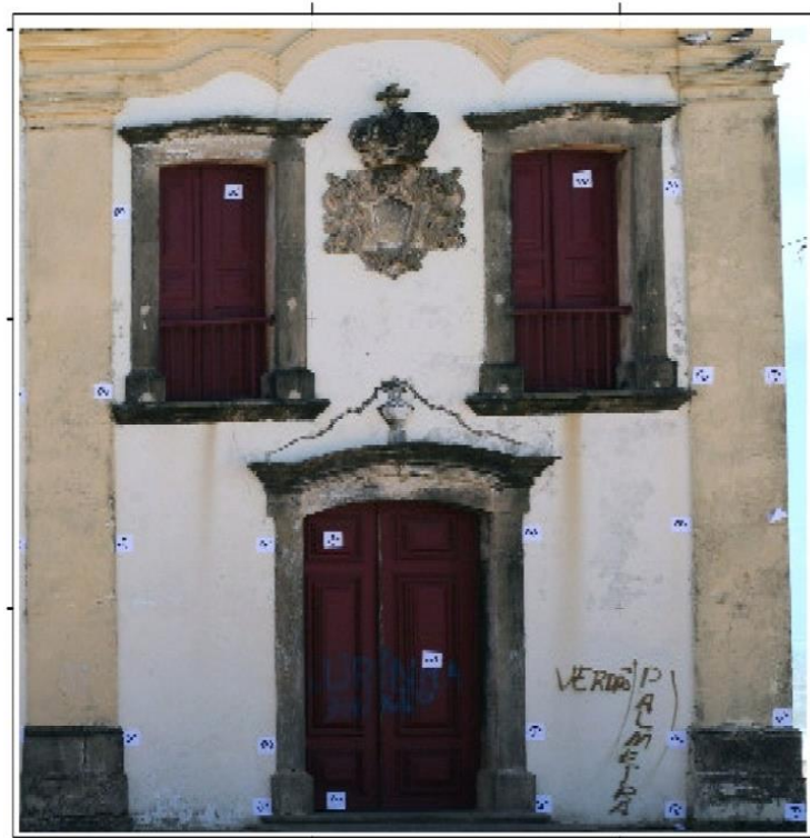
Figura 28: Ortofoto gerada no PhotoModeler Scanner
