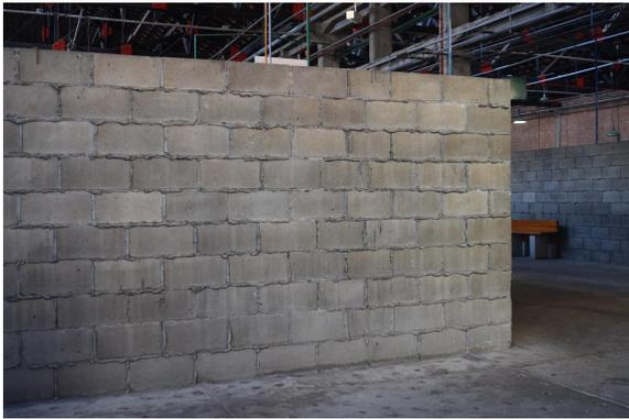
**Fig. 22: PAREDE DE BLOCOS COM ARGAMASSA.**
