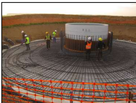
(a) Foundation under construction.
