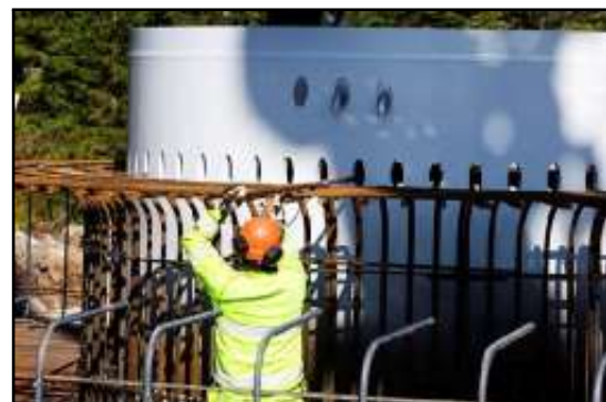
(b) Detail of longitudinal bars crossing the ring wall.
