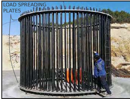
(a) Anchor bolts cage.
