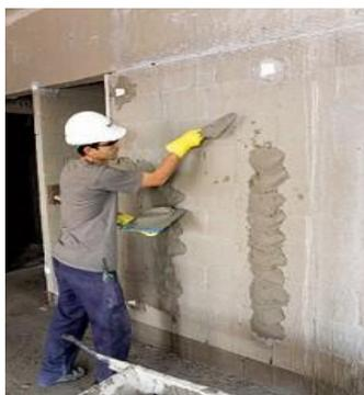
Figura 3 – Reboco manual
