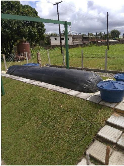
Figura 14. Biodigestor experimental de 8m<sup>3</sup>
