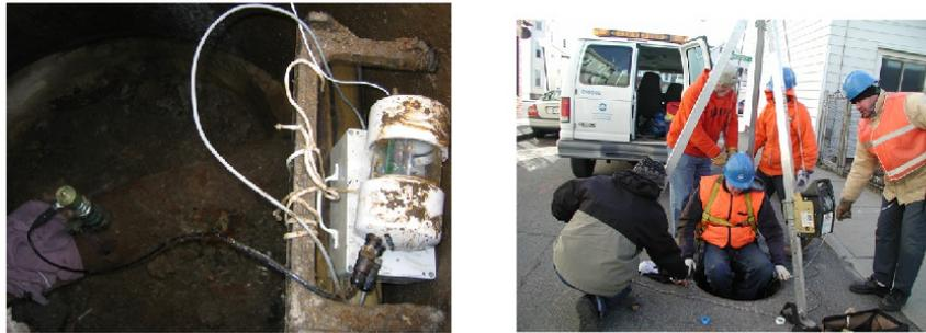
Figure 10: Cluster 2: Installation of the pressure sensor node
