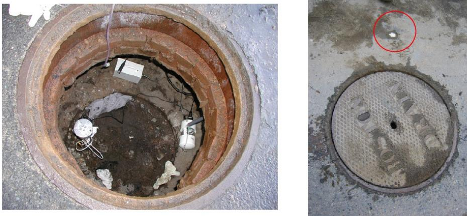
Figure 9: Cluster 1: Installation of pH probe; Antenna embedded in the road surface
