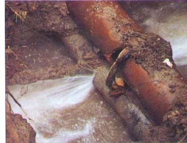
Figure 3: Leaking water and sewer pipes (Courtesy of AWWARF)
