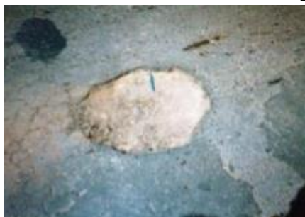
27(a) Panela atingindo a base (P)
