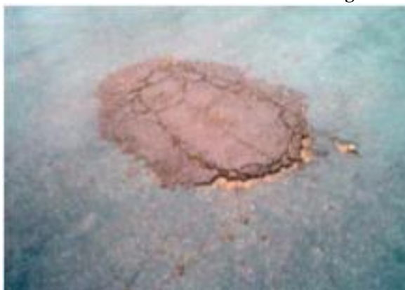
28(a) Remendo mal executado (R)
