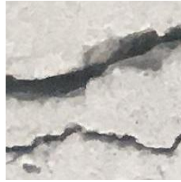
Figure 3 - Example of a concrete crack image containing two cracks.
