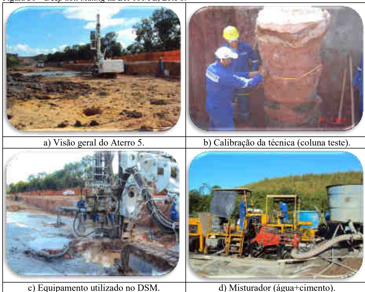
Figura 30 – Deep Soil Mixing na BR-101/PE, Lote 6.
