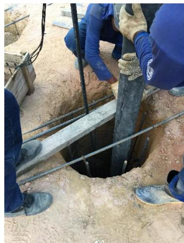
**Figura 118 – Estacas concretadas**
